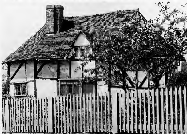
TWO TIMBERED COTTAGES IN KENT COUNTY
